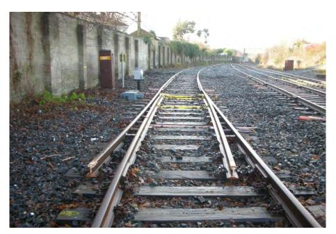
Figure 4-211 Current siding trap point. Source IAMS
