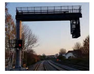
Figure 4-12 Sample cantilever signal gantry
