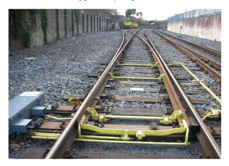
Figure 4-210 Current siding P10-10 turnout. Source IAMS
