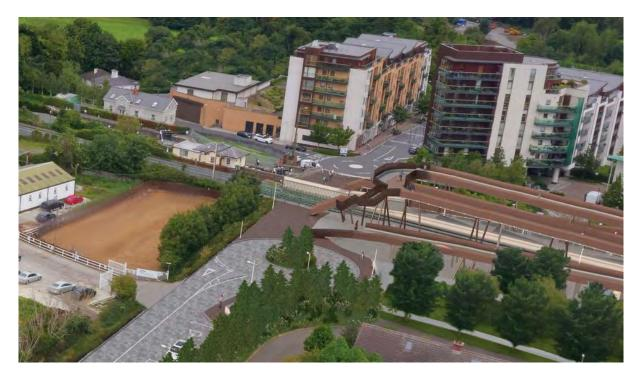
Figure 4-141 Ashtown Station after removal of level crossing
