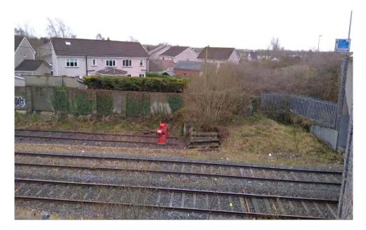
Figure 4-212 Current siding buffer stop. Source IDOM
