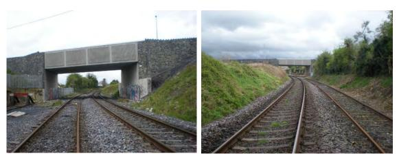
Figure 4-215 Left: siding to be converted into a running line. Right: siding with wood sleeper and without cant
