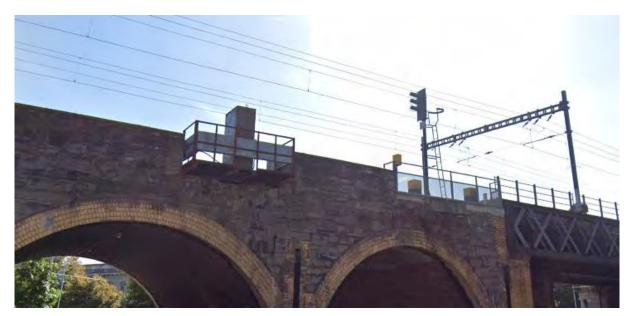
Figure 4-14 Signalling equipment installed on a bridge platform.
