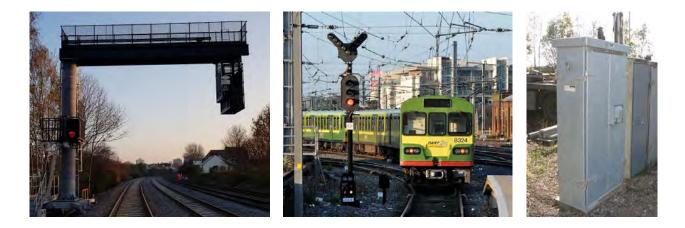
Figure 4-10 Sample DART+ West signalling infrastructure (cantilever, signal, LOC, from left to right)
