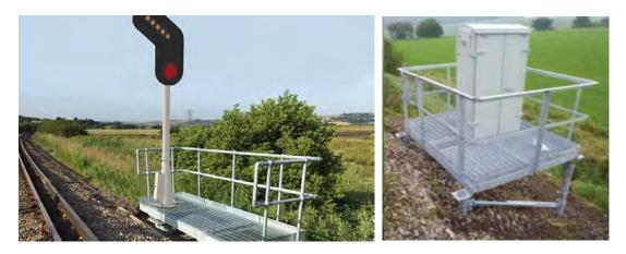
Figure 4-13 Signal and LOC installed on a platform
