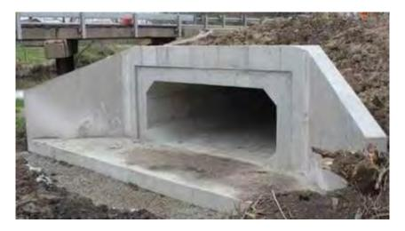
Figure 4-259 Indicative flood relief culvert
